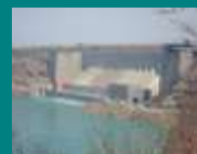
Niagara Power Plant Lewiston, NY
