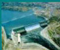
Grand Coulee Dam, Coulee City, WA
